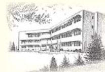
Lawrence Memorial Hospital 1980-1999
